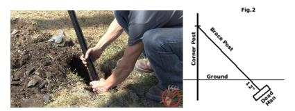
Dig a hole 1' deep where the brace post contacts the ground. Place a dead man (cinder block, large brick, or stone) in the hole perpendicular to the brace post. Wedge the brace post against the block to provide support for the vertical end post.
